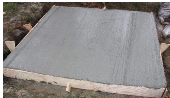
Fig. 1 Casting of the steel-fibre reinforced concrete slab
